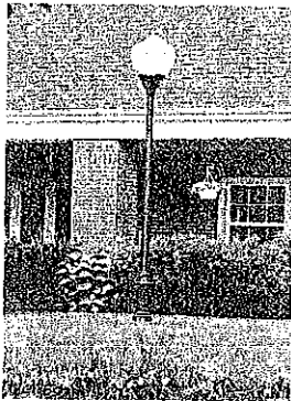
This light standard is somewhat traditional but equally as popular. Its overall height is sixteen feet. The light source is mounted on a cast aluminum post that closely simulates cast iron. The light globe is made of opaque glass to diffuse the light source and reduce glare.
